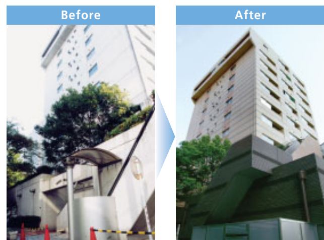
Originally constructed in 1981, Palms Gotanda in Shinagawa Ward was restored to newly built condition through complete renovation of all common areas, including facades, entrance and exterior.
