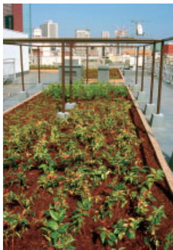
Takanawa Tosei Building, Minato Ward
