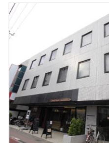
Hlno-shi Income-generating Building
