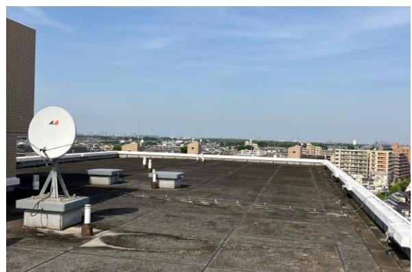
Rooftop where solar panels will be installed
