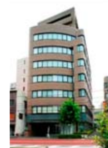
Ueno Takeuchi Building
