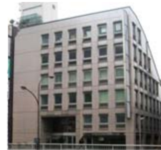
Rosebay Shinjuku Building
