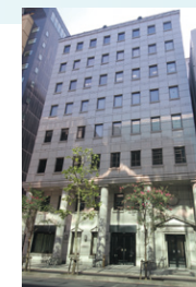
Hatchobori Tosei Building III
