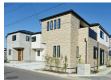
THE PALMS COURT Tsunashima (detached house series)
