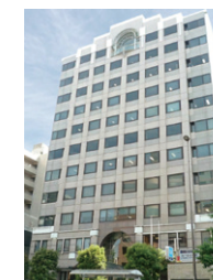
Narimasu Tosei Building
