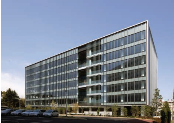
Heiwajima Tosei Building
