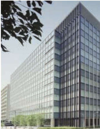
Kamata Tosei Building
