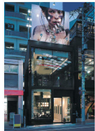
The Shinjuku Shogyo Building in Shinjuku Ward, Tosei's first commercial development project, takes maximum advantage of its location.
