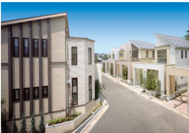
THE Premium Court Ota Chuo residential subdivision in Ota Ward features 43 large-scale lots on a south-facing slope.
