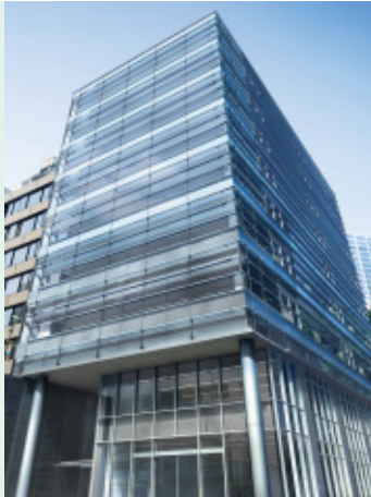
Toranomom Tosei Building, (Minato Ward)
