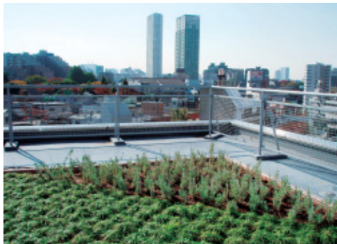
Takanawa Tosei Building, Minato Ward
