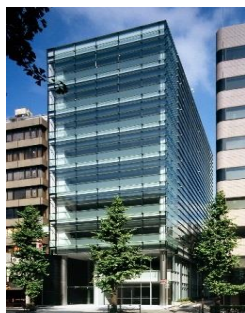
Toranomon TOSEI Building
