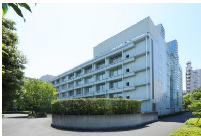
Nishidai Tosei Building
