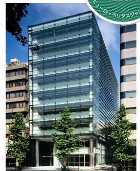
Toranomon Tosei Building
