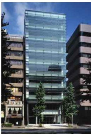
Toranomom Tosei Building
