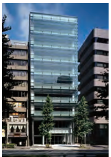
Toranomon Tosei Building
