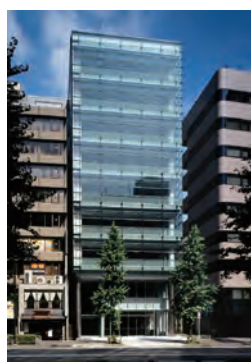
Toranomon Tosei Building
