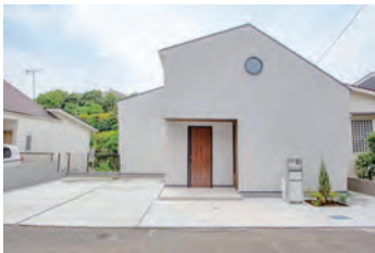
Example of ZEH construction
