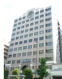
Narimasu Tosei Building
