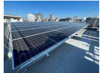
Solar panels installed on the rooftop
