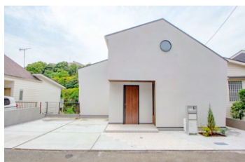
Example of ZEH construction
